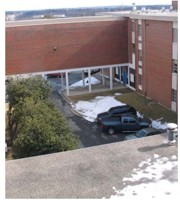
Southeast Entrance Lobby
