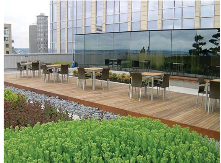
A green roof offers superior insulating vaues while reducing storwater run-off
