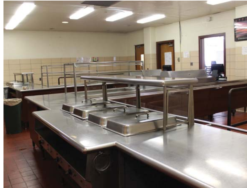
Existing Serving Line
