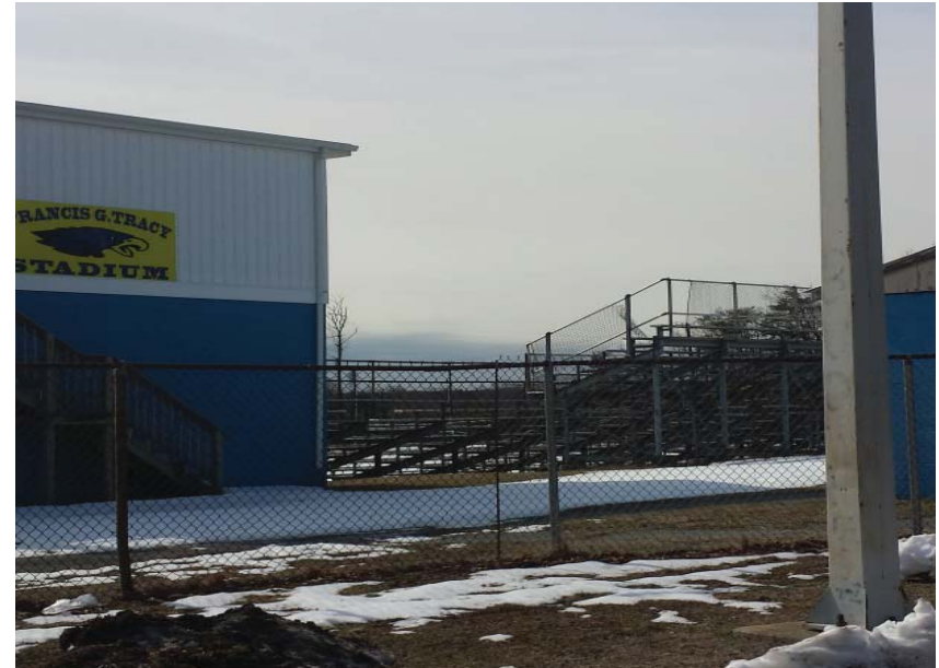
Existing Football Field/ Track and Non-Accessible Stands
