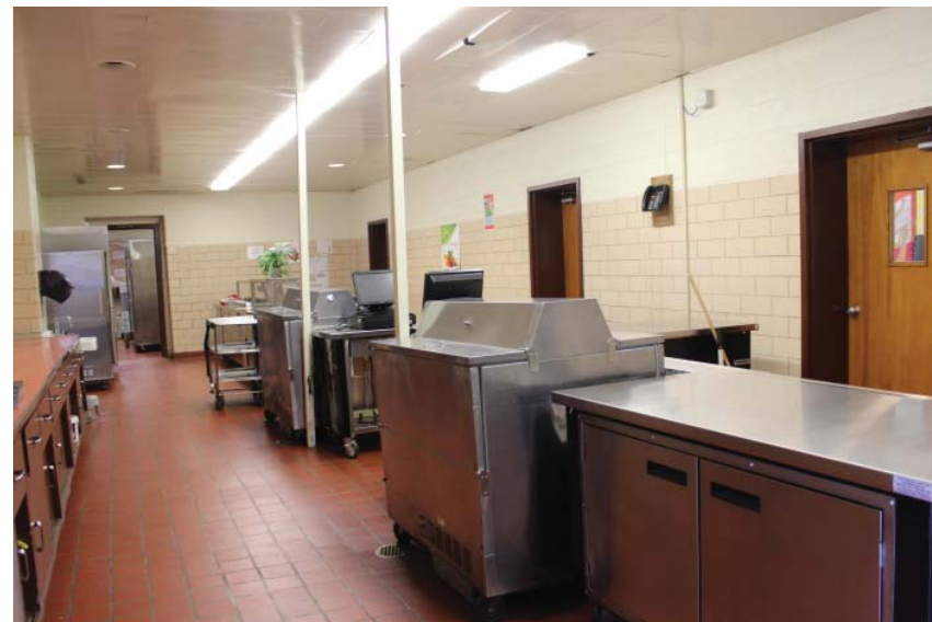
Existing Serving Line
