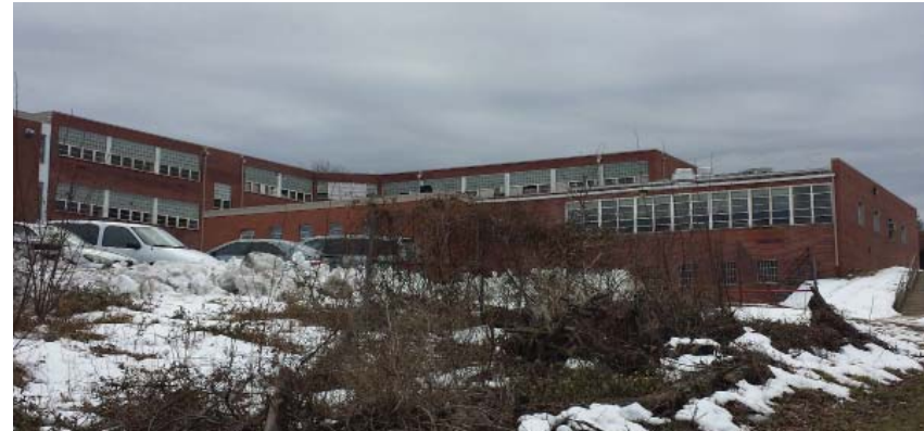
View of Northeast Parking Lot as Approaching School From Eastside
