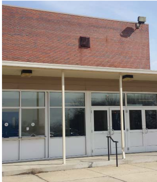
Entrance at Gym
