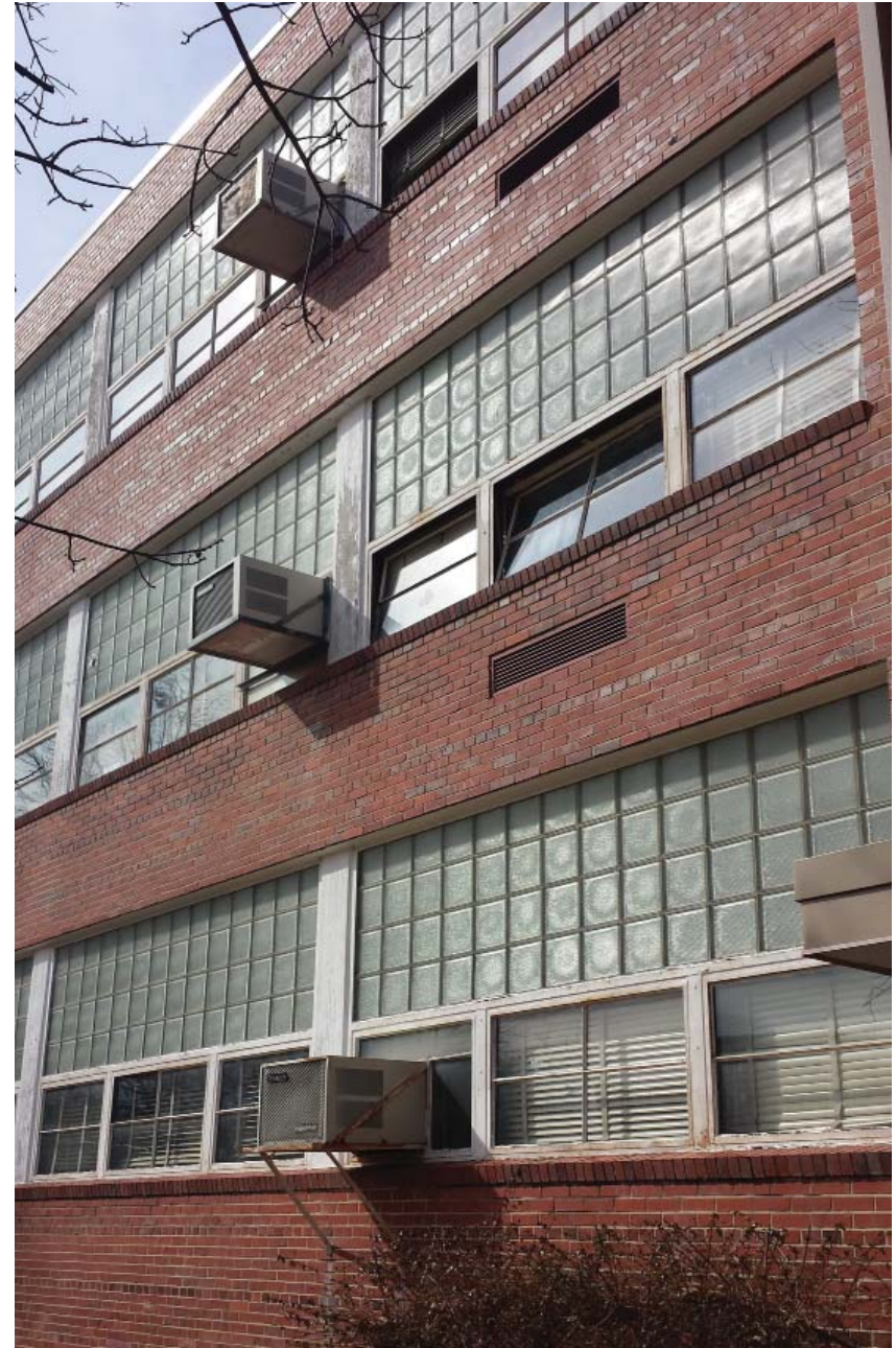
Existing masonry and glass block exterior wall
