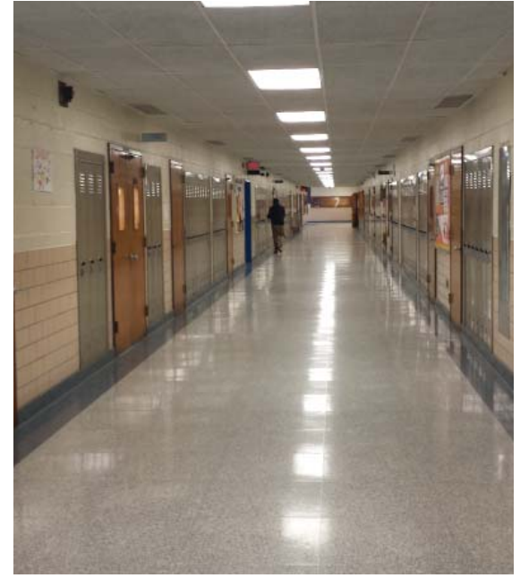
Administrative Wing Corridor
