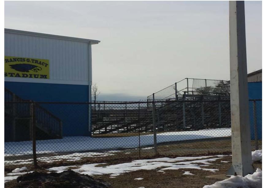
Existing Football Field/ Track and Non-Accessible Stands
