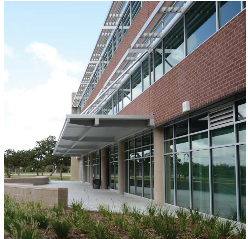
College Satation High School, College Station, Texas - South Facade Sunshades
