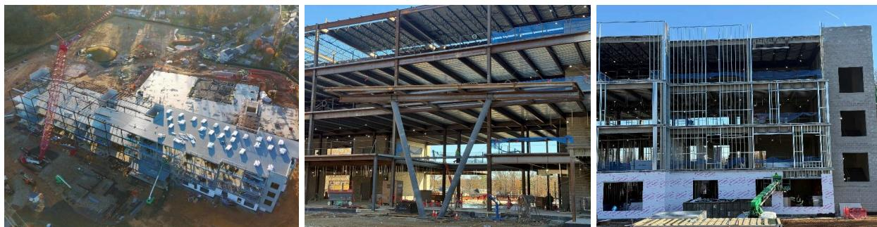
Construction has made significant progress at the Robert Frost K-8 site. This past quarter, the construction team completed asbestos abatement, interior demolition, and full raze of the existing building. Rough and final grading, building foundations, Phase 2A and 2B storm drain installation, below-grade masonry, and the relocation of storm and sewer lines, managed by WSSC, were also
