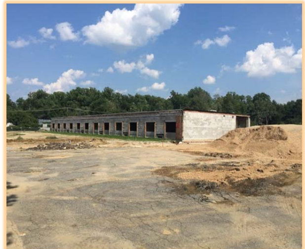
Tulip Grove ES Completed Demolition
