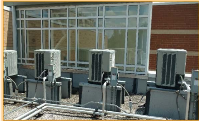
Roof Top Unit Replacement
