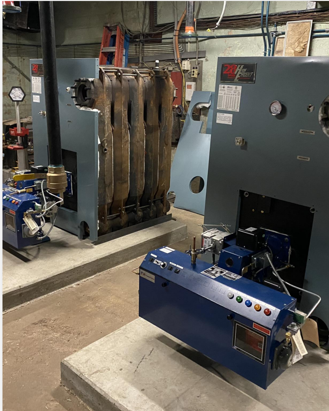
Hollywood ES Boiler Replacement
